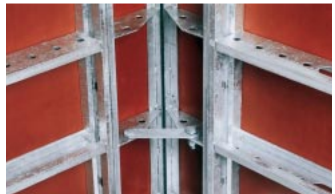
above: Outer corner clamps and two normal panels form the outer corner. They also facilitate length adjustments of 4 to 6 cm below: The inner corner has 2° of clearance for easing
