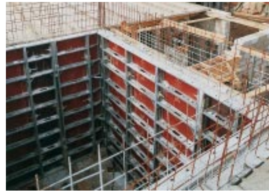
above right: Adjacent panels are held with a single tie below middle: Stopend with the MANTO-multi-purpose waler and centering tension bolts
