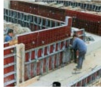
Interior tie pockets enable panels to be used on their sides without supplementary aids
