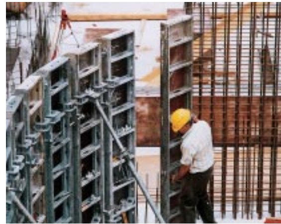
Interior tie pockets enable panels to be used on their sides without supplementary aids
