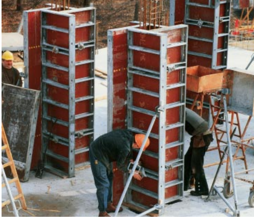
Column formwork with RASTO-multi-purpose panels. Columns can also be shuttered with standard panels and outer corner clamps
