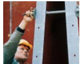
middle right: Panel connections simplified with the centering tension bolt
